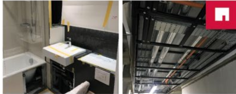
Category 5a. and 5i. MMC – Mace for QDD at East Village
