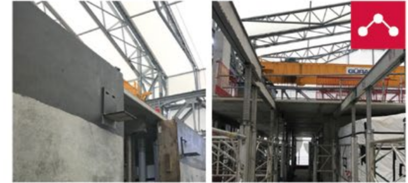
Category 3c. and 3d. MMC – Mace for QDD at East Village
